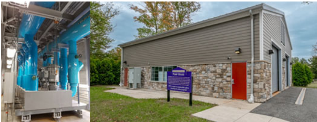
WCU Geothermal Central Distribution System
